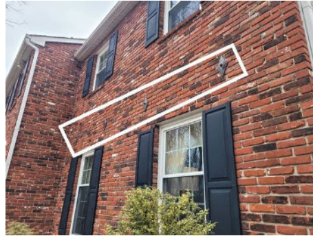
Note four anchors
