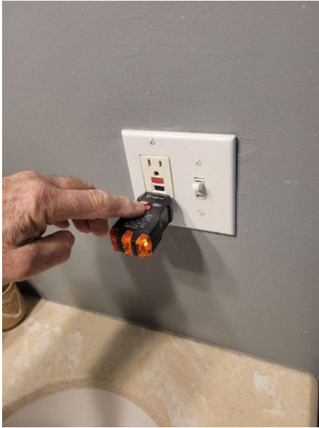
location is primary bathroom
